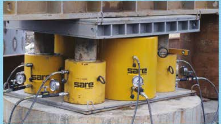
STATIC PILE TESTING JACKS
